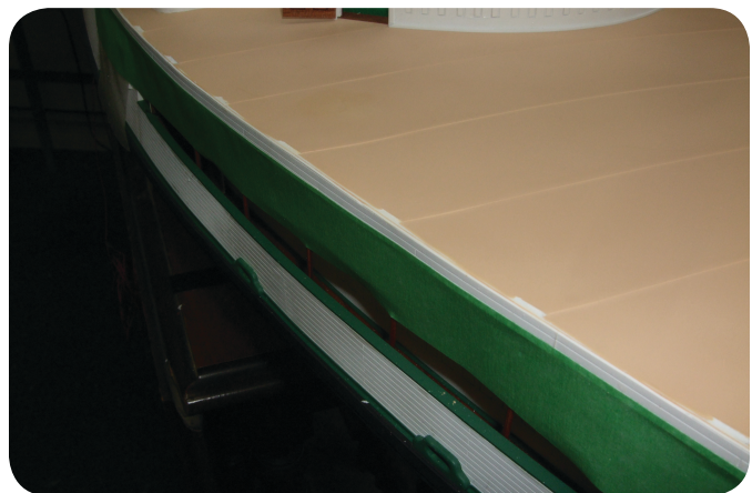
Photo 291. The simulated canvas deck must be carefully removed at the edges to accommodate the water boards.
