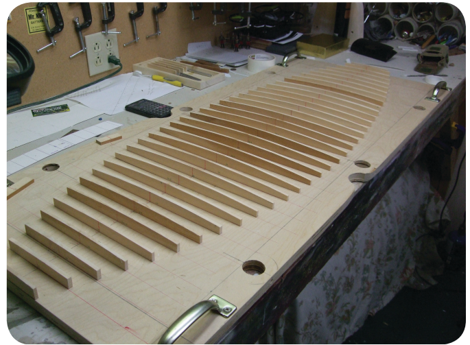
Photo 256. The building board jig was created to ensure that camber would be consistent over the entire first deck surface.
