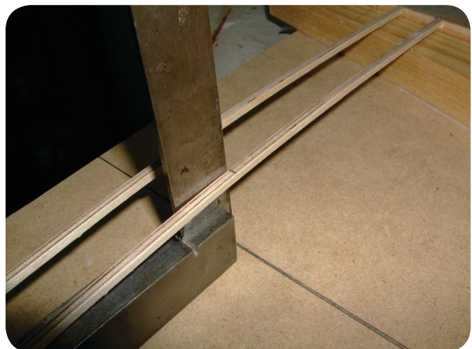
Photo 177. A square was used to align the center of each ceiling beam to the center of the form. The ends were cut from each ceiling beam so that they would fare into the side beams.
