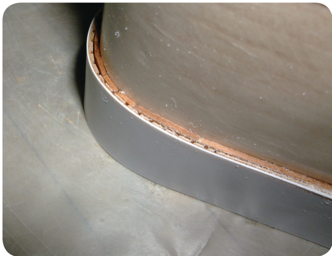
Photo 113. The plywood laminate was relief cut to allow it to conform to the curve.
