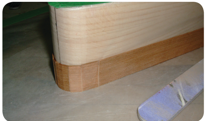
Photo 112. The cherry wood laminate has been attached to the plug by two sided tape.
