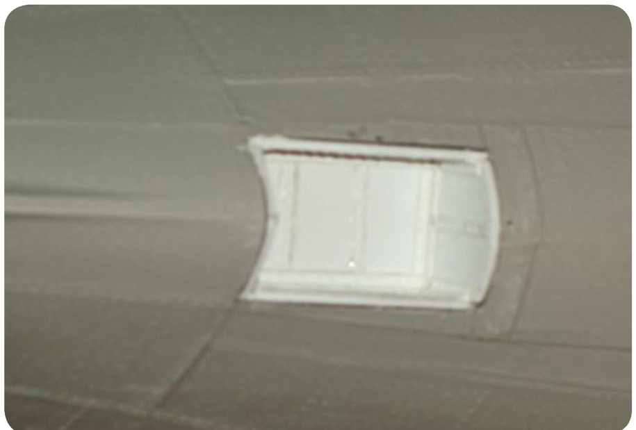
Photo 4. Asdic well detail.
